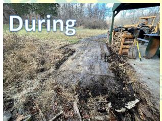
The area was scraped with the backhoe and back filled with crushed run. This new area is perfect for troop trailers with easy access from the shelter. The johnny blue was moved to the other side of the shelter and the area to the
